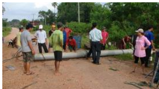
Local villagers remove the PVC headwater pipe
