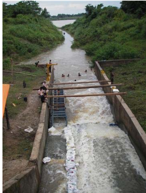
Upstream view of the fishway. The sandbag wall was used to control flows through the structure
