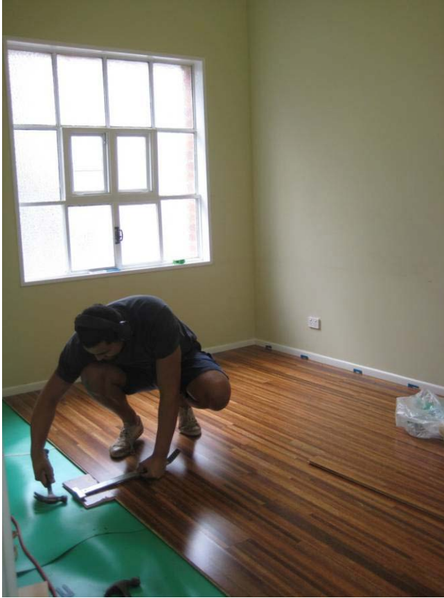
Plate 10. Engineered cocowood flooring installation, Brisbane.
