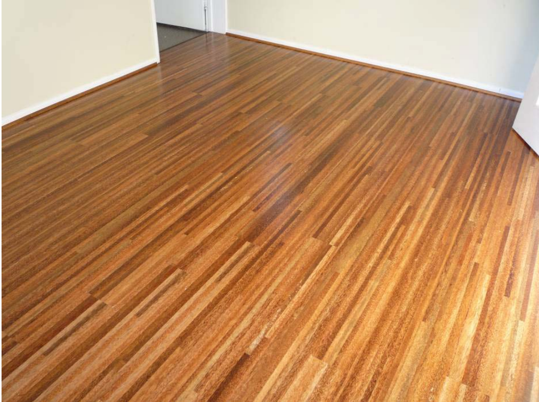
Plate 12. Engineered, pre-finished cocowood flooring in service, Brisbane.
