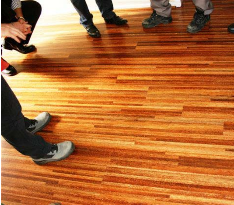
Plate 11. Feature flooring- engineered cocowood installation, Brisbane.
