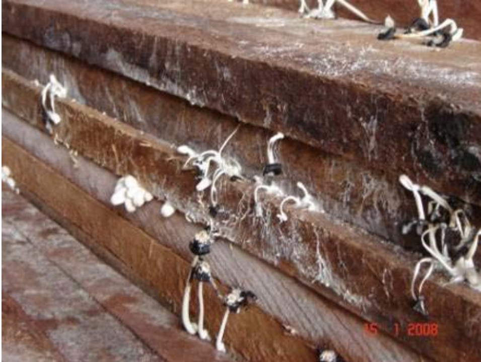
Plate 11. Fungal fruiting bodies growing on untreated cocowood boards.
