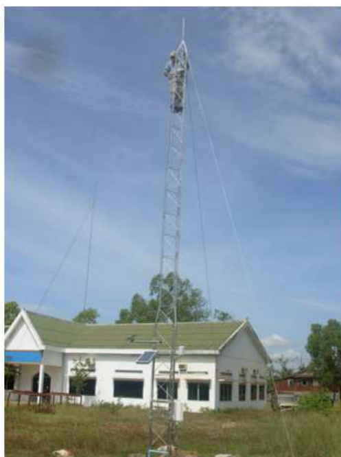
Figure 5-8 Installation of weather station at the Takeo MOWRAM field station
