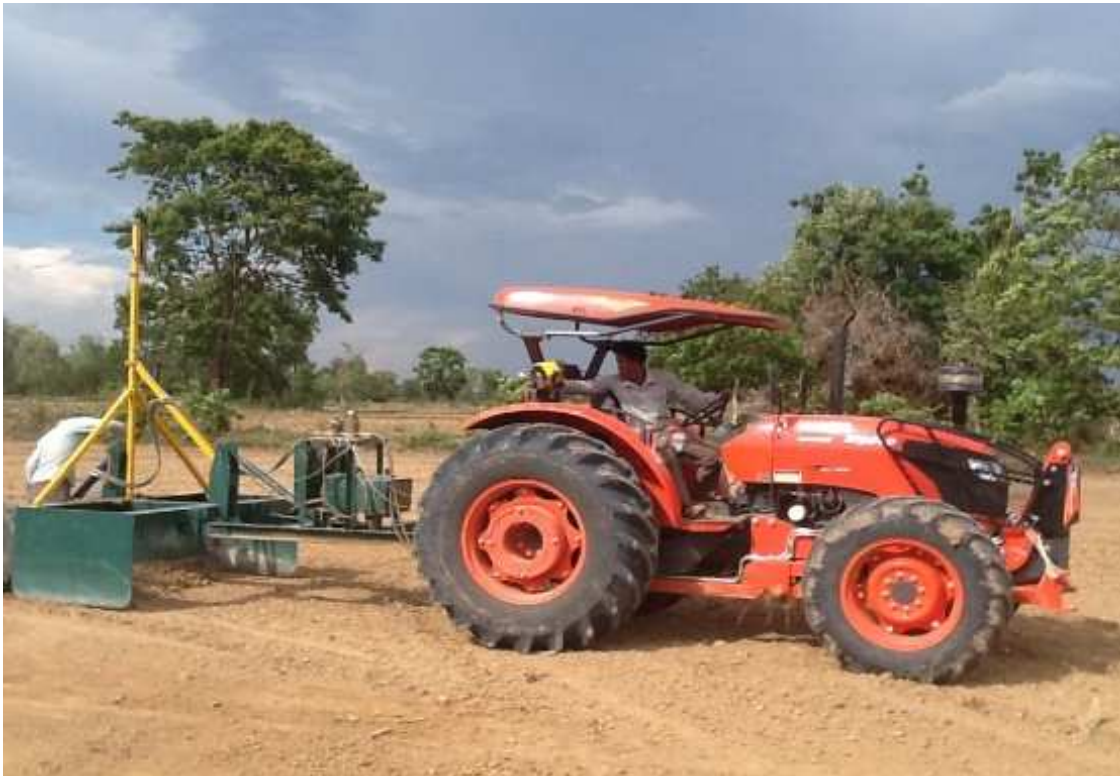
Figure 7-38 Contractor operating in Battambang Province with levelling equipment and 95 HP Kubota
