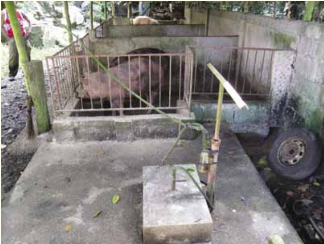
A smallholder biodigester in Eastern Leyte using pig effluent to produce biogas for household and neighbourhood use.
