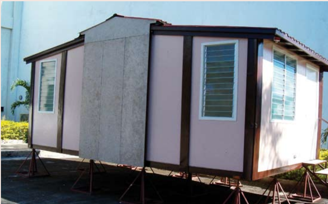
Emergency, foldout shelter prefabricated from wood-wool cement-boards, Forest Products Research and Development Institute, Los Baños, Philippines.
