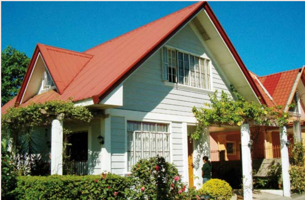
Home built almost entirely out of wood-wool cement-boards, Quezon city, Philippines.
