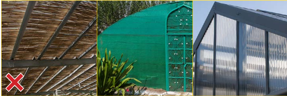
Figure 2.6 Materials for covering plant houses include lath (not recommended, left) shade cloth (centre) and polycarbonate (right).
