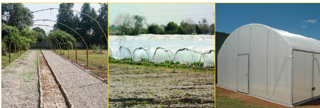
Figure 2.5 Quonset plant houses. In Pakistan, quonset plant houses are often made with bamboo frames and covered with plastic (left & centre). Modern quonset plant house frames in commercial nurseries are often constructed with light-weight aluminium (right).
