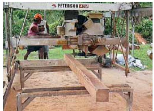
High density boards removed
