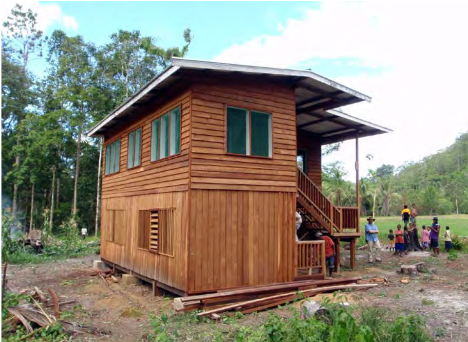
The Sogi community has constructed a community house from locally milled kwila in Yagi village (Photo: Julian Fox).
