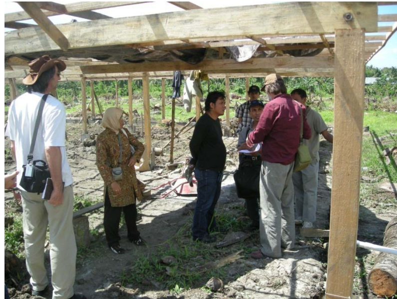
Fig. 4 Nursery under construction in Padali, Soppeng
