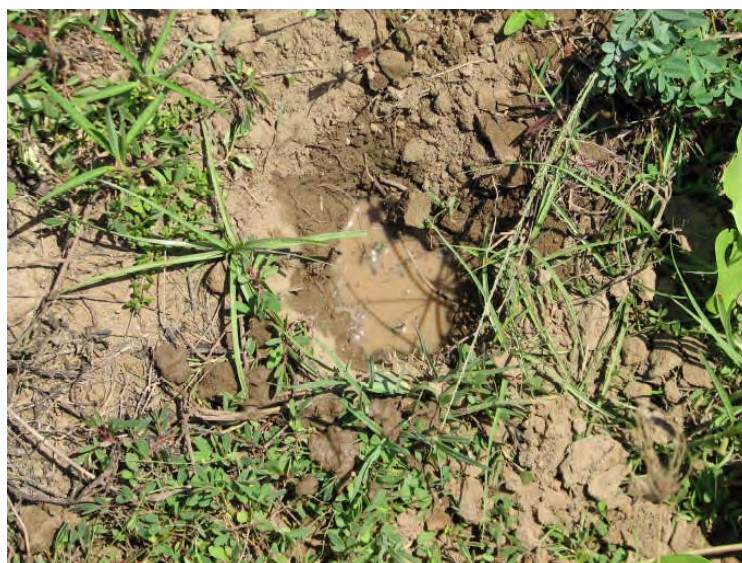
Figure 6. Poor water infiltration was observed in a derelict vegetable field near Kling Cot Arun village in Baitussalam Sub-district, Aceh Besar District.
