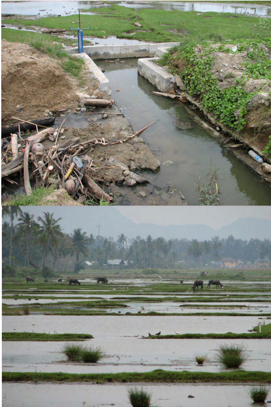
Figure 3. The tsunami damaged irrigation and drainage infrastructure (top) making it difficult to deliver irrigation water and drain lowland rice and vegetable fields, which remain derelict (bottom).
