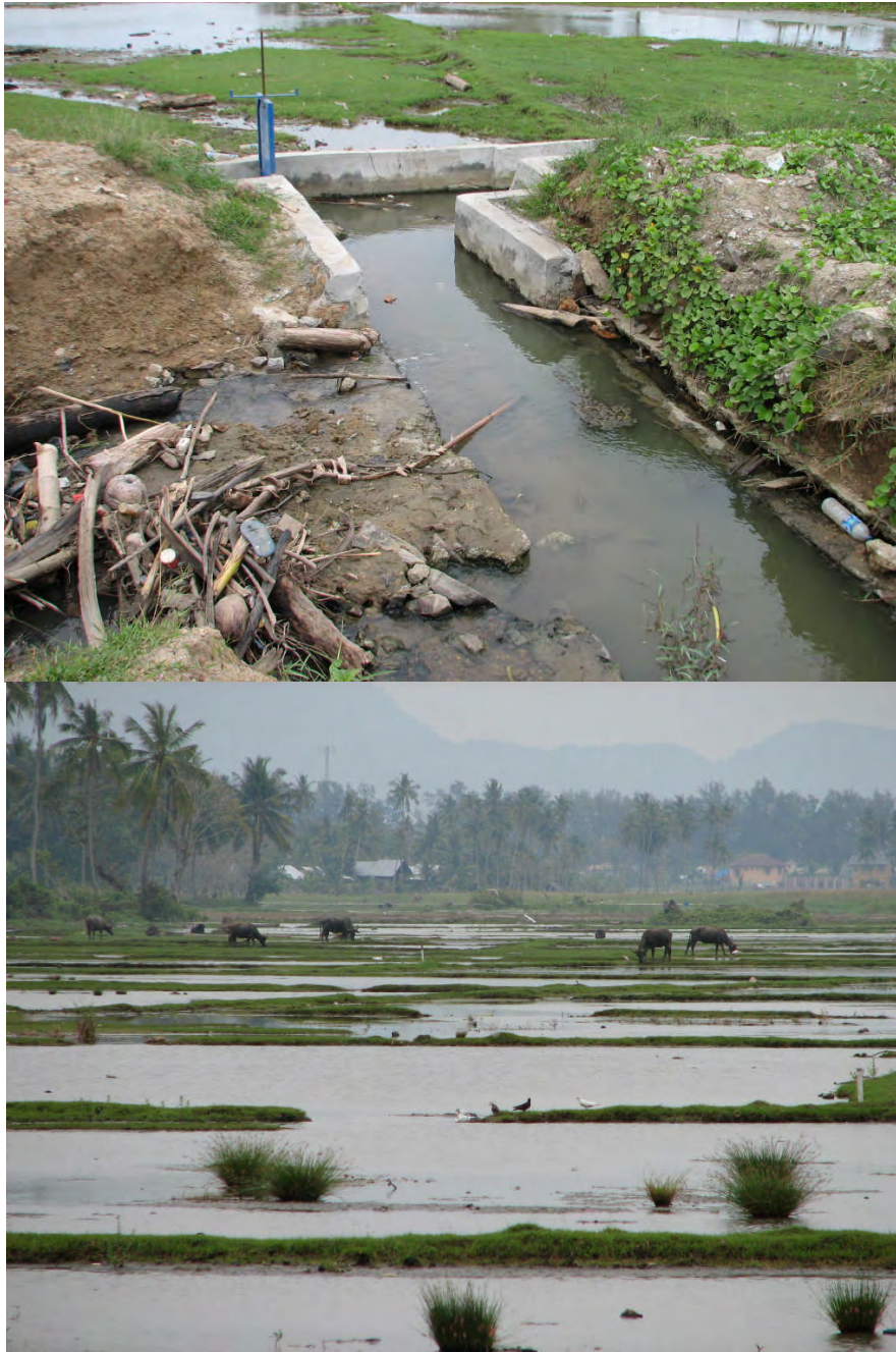
Figure 3. The tsunami damaged irrigation and drainage infrastructure (top) making it difficult to deliver irrigation water and drain lowland rice and vegetable fields, which remain derelict (bottom).
