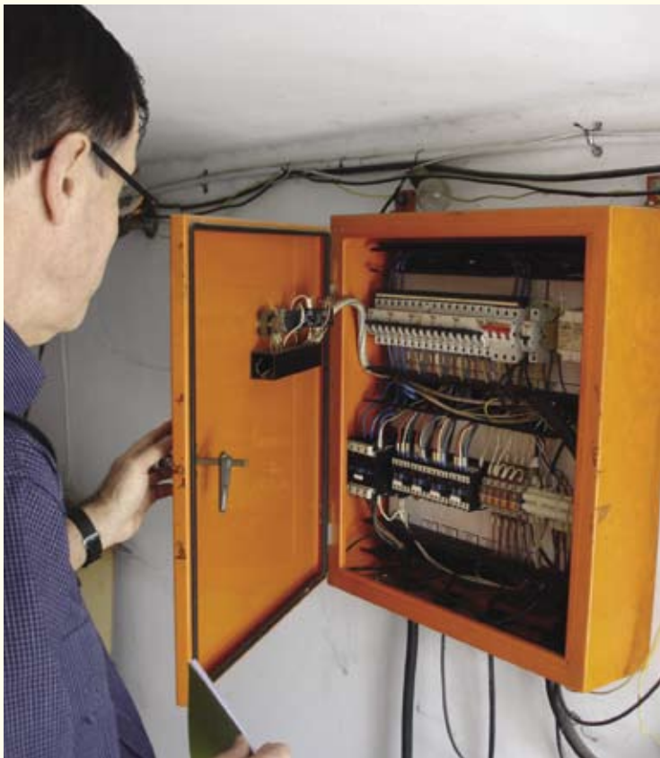
Australian project scientist Dr George Srzednicki confirming the status of an aeration control box after installation at Zhaodong grain storage depot.
