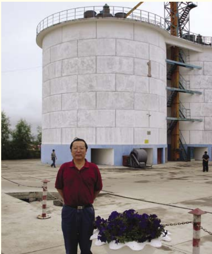
Liu Fangjiu outside Zhaodong converted storage silos, showing the large intake of the aeration fan which feeds the internal vertical aeration piping.
