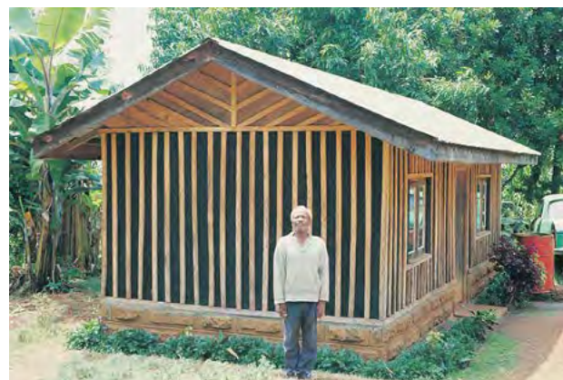
House constructed using G. robusta timber; Kenya (Photo: CSIRO)
