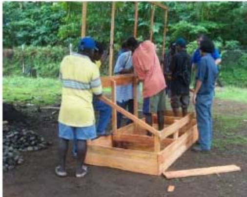
Building the frame for the poly-propagator.
