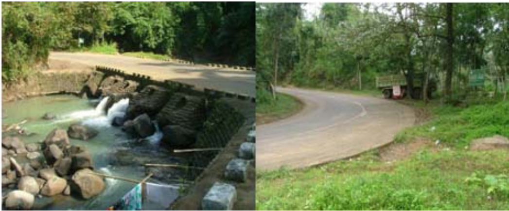
Figures 10 and 11. Equipment was initially installed near the Brangay Tibatib Overflow Bridge at Cavinti just beyond the green sign in the right-hand photo.
