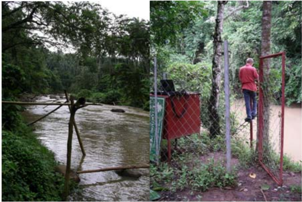
Figures 12 and 13. Autosampler and waterlogger on the Bongbongan River at Caviniti.
