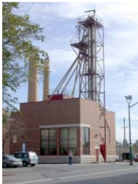
A view of the research facility showing two storage bins and two bucket grain elevators.
