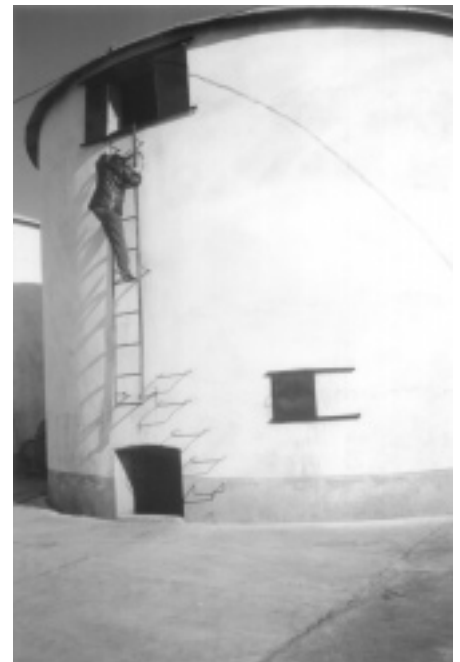
In-store drying experiment at the Sifang Grain depot in Zhaodong, Heilongjiang Province: Dr Niu Xinghe inspects the grain silo.
