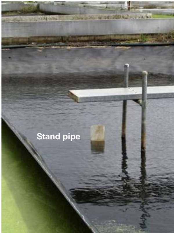
Figure 5. The internal standpipe, the top of which is 10 cm below the water surface, taking the water to be returned to the fish pond from the surface of the treatment pond. The water level has been lowered to allow the stand pipe to be exposed for the photo.
