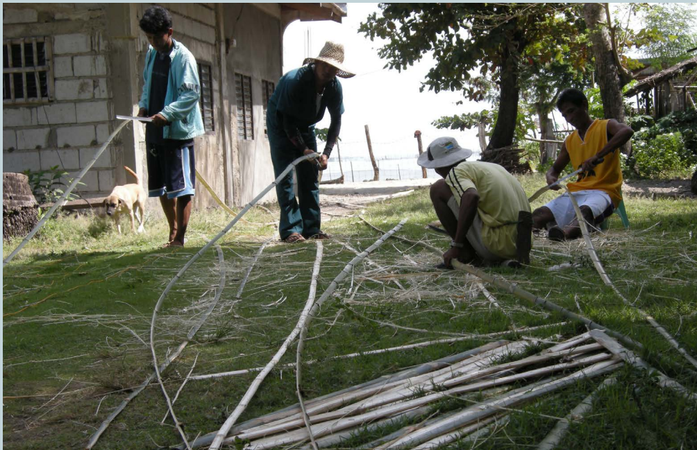
Figure 17 Pen construction for the Sablig sea ranch
