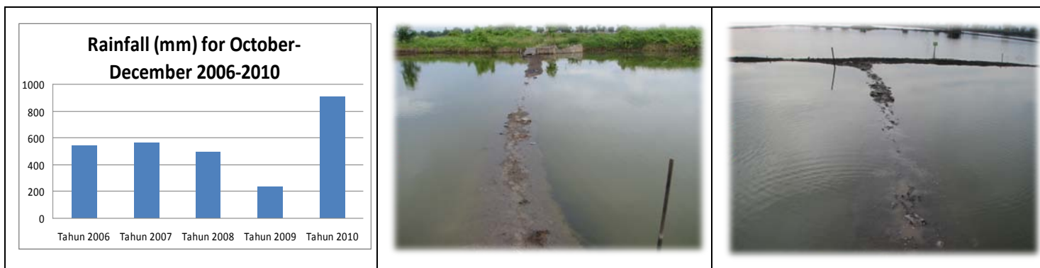
Figure 15. The entire site was flooded in November 2010. Left: Graph showing last-quarter rainfall (mm) for years 2006-2010 at Kendal; centre and right: typical partly submerged pond embankments.
