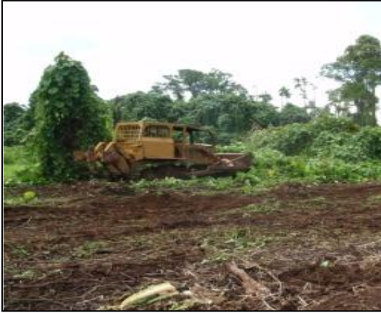
Figure 25 Using large tractors to clear a site prior to planting.
