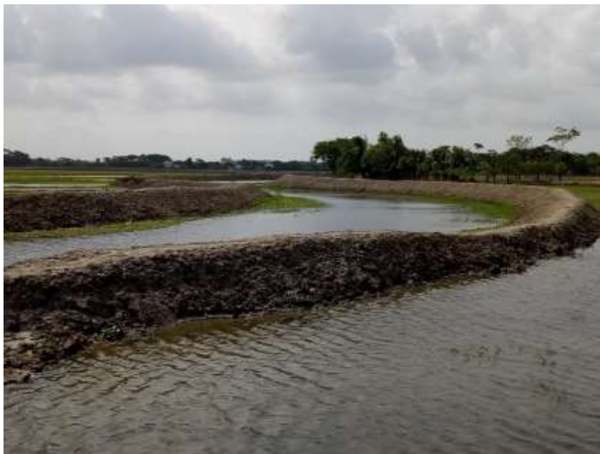
Figure 8.5 Re-excavated canal at Amtali. At the top corner there are rice field (Aus rice) grown using canal water.
