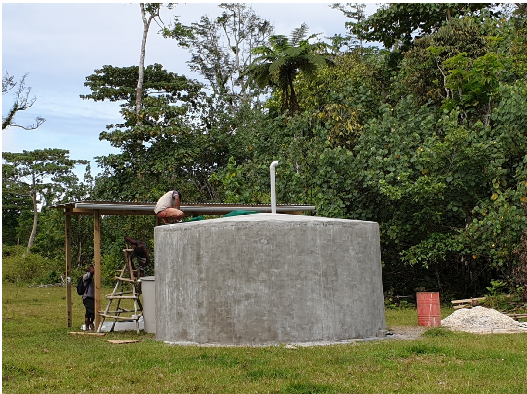
Figure A2.21. Cement water tank and catchment established near Port Olry, East Santo Area Council.
