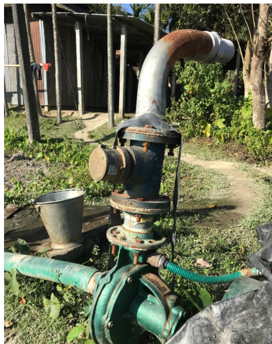
Figure 32 Flow meter installed too close to the pump and a pipe bend
