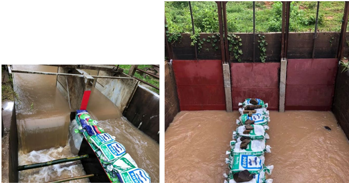
Figure 23. A sandbag wall was installed to separate the left and right gates, thus enabling two gates to be independently trapped at a time.
