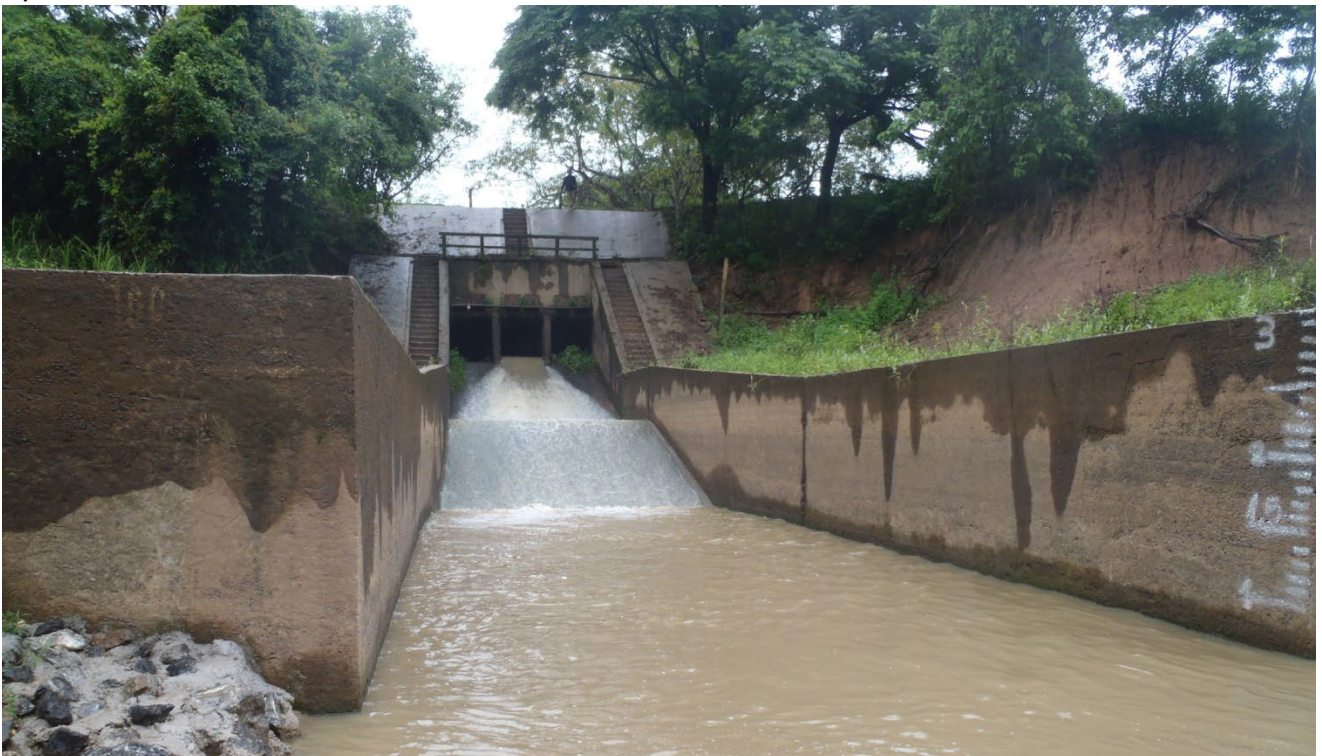
Figure 3. Pak Peung Regulator a) viewed from the upstream direction showing the three ‘undershot sluice gates,’ and b) from the downstream direction at the onset of the wet season. In a typical wet season the Mekong River will rise so that the box culverts become submerged.
