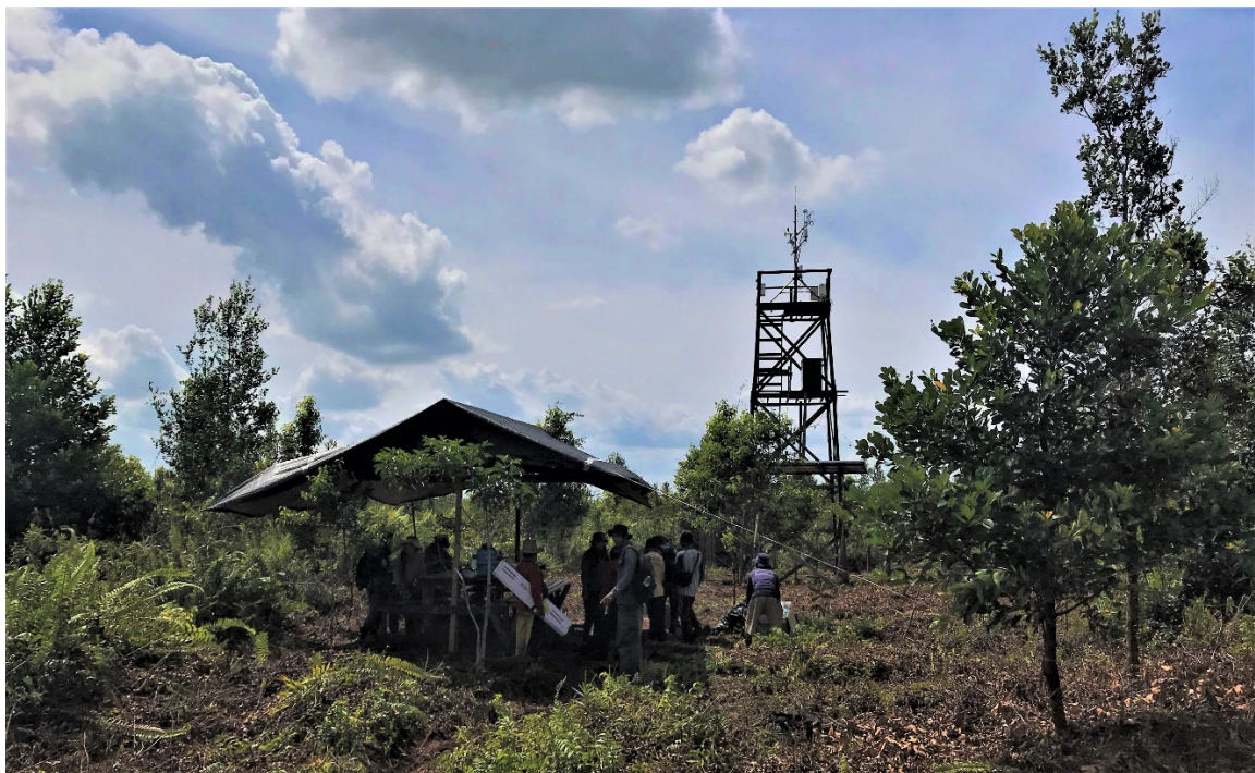
Figure 1 The project team onsite during the flux tower and Chameleon sensor installation, July 2019. The flux tower consists of an 8 m platform with gas analysers and wind speed sensors mounted on the upper platform. A 110V AC / 12 V DC solar system provides reliable power the system.
