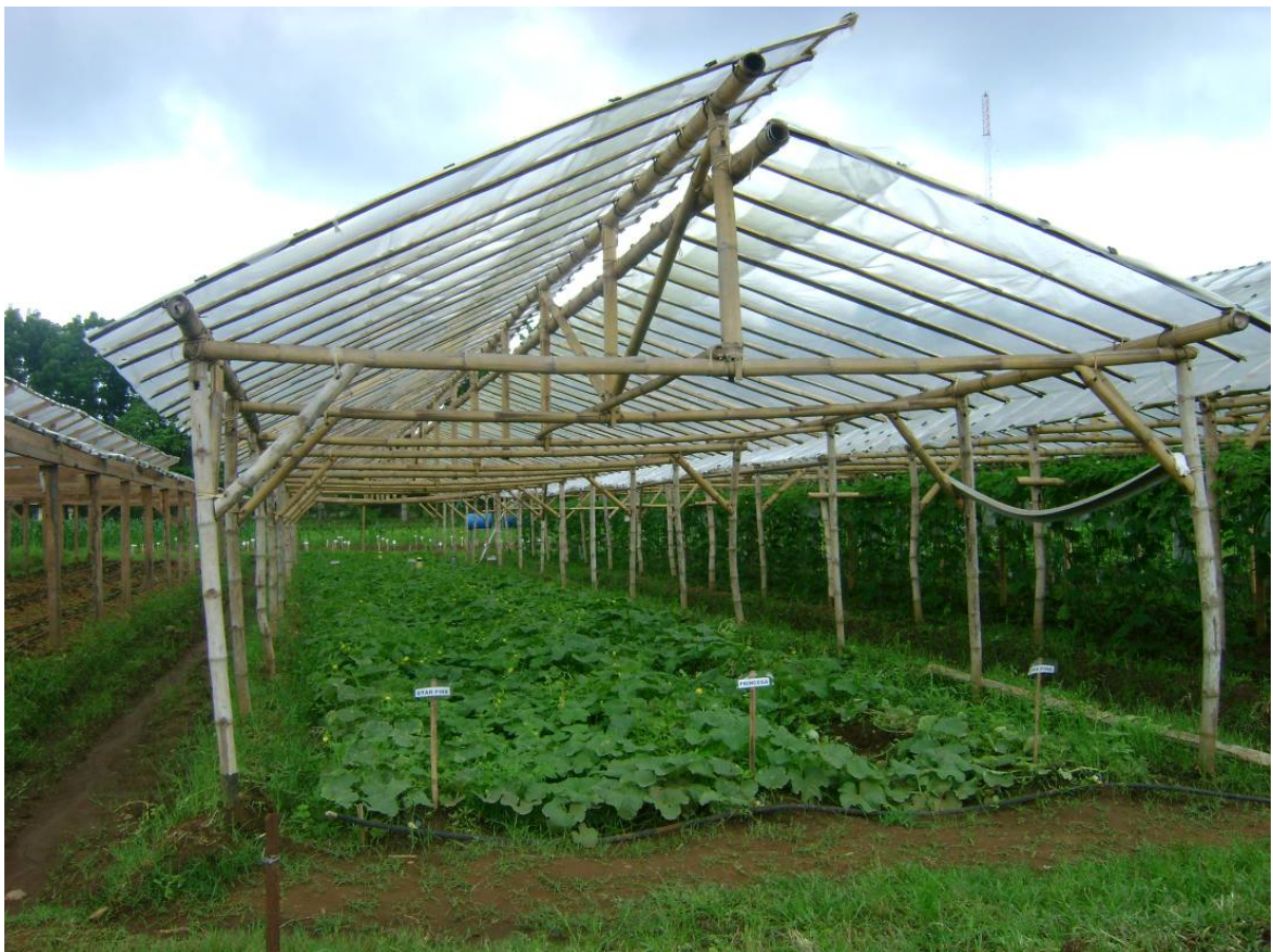
Photo 1. House type structure made of Bamboo
