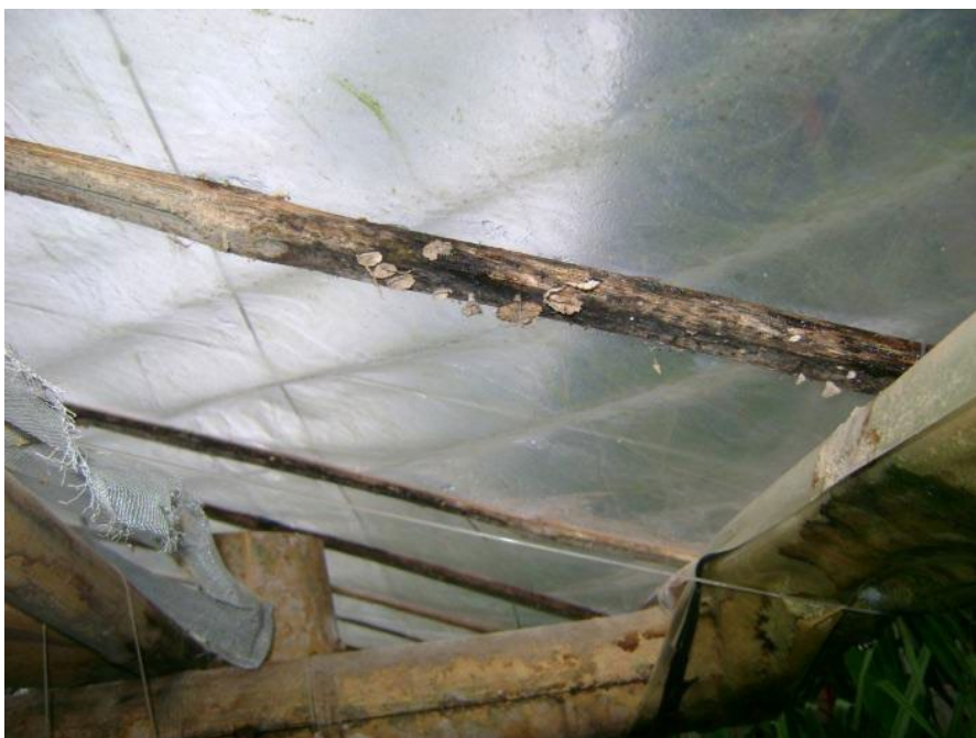
Photo 11 Damage to bamboo from water leaking
