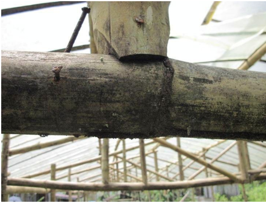
Photo 10 Termites attacking the bamboo
