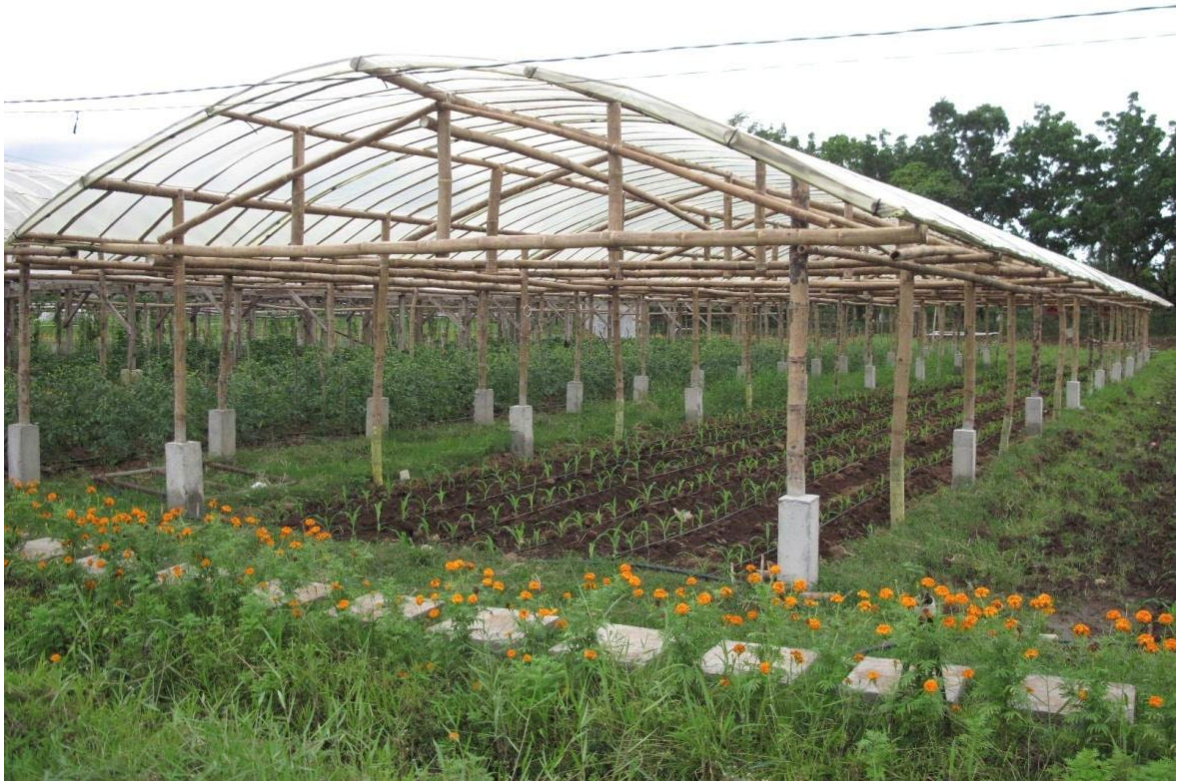
Photo 4. New curved roof design (with sides enclosed)
