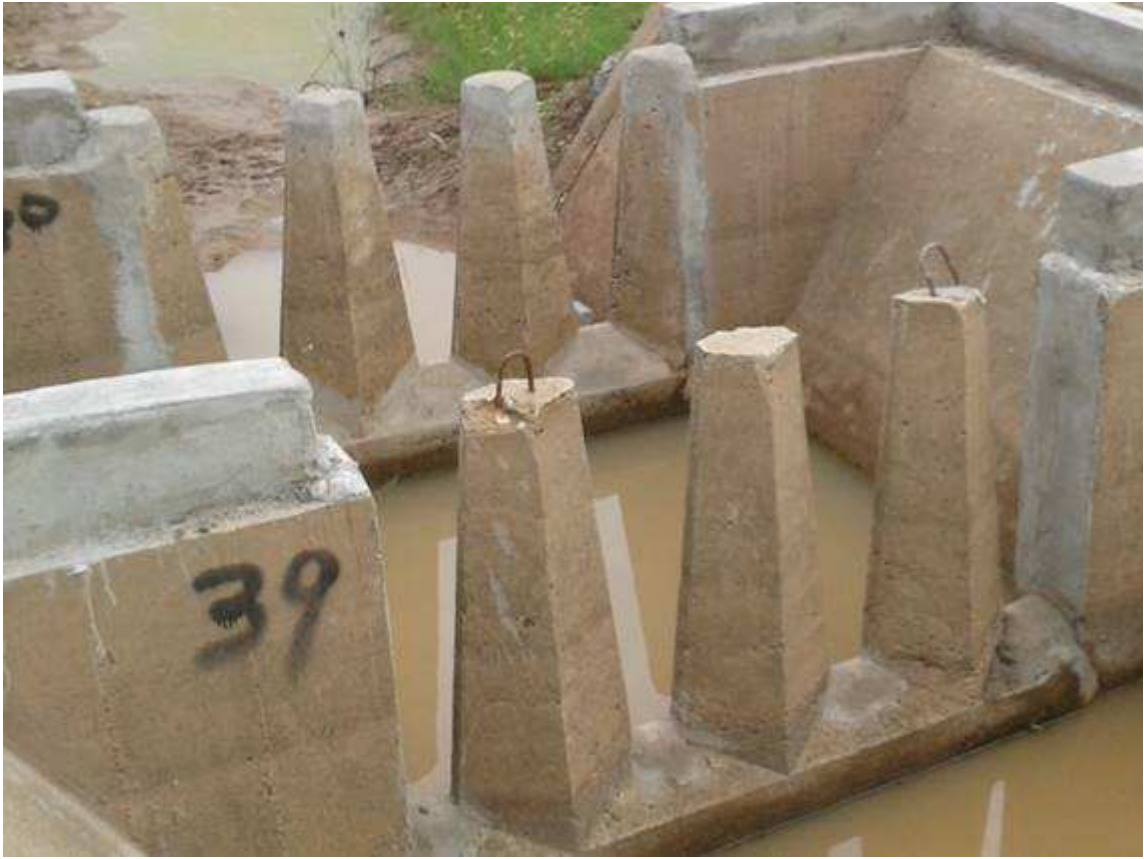
Figure 6. Alternating concrete cone baffles with three full slots (background) and two full slots and two half slots (foreground).
