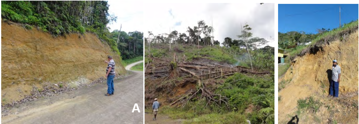
Plate 15 Deep colluvial soils are common on the hillsides on the road to Tapini (A), food gardens are created by slash and burn on deep colluvial soils (B), deep colluvial soils at Tapini village
