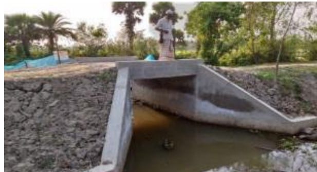
Image 6 Hafamari canal after re-excitation in July 2018, left and newly constructed culvert to channel freshwater in 2019, right
