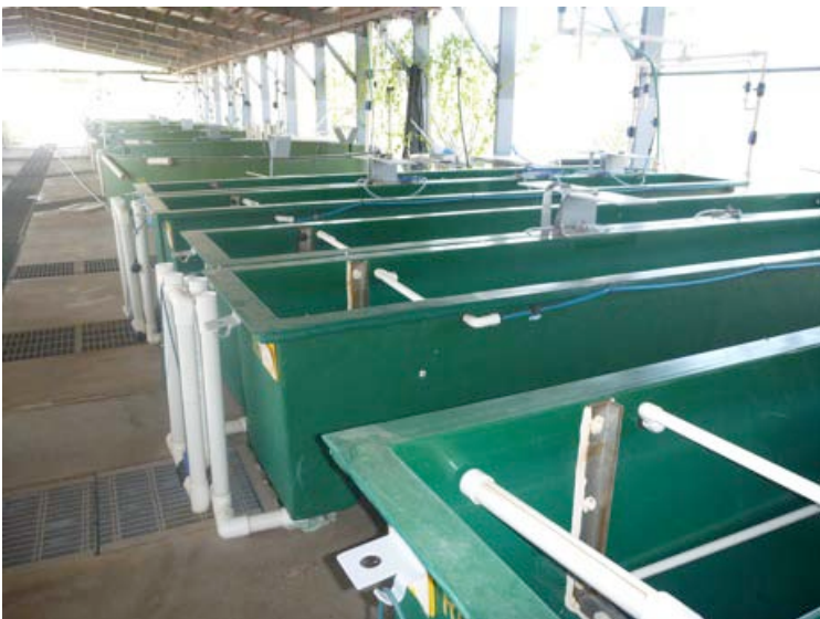
Figure 5: Typical raceway tanks in Darwin, Australia
