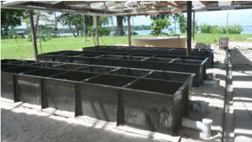
Figure 4: Raceway tanks at Nago Island, PNG
