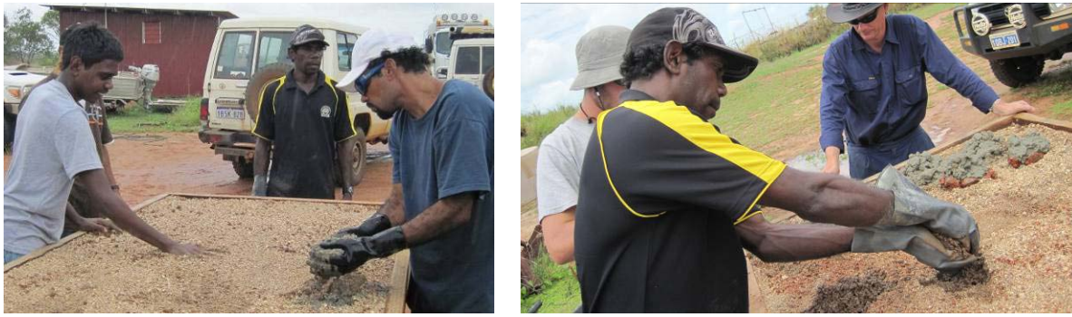
Figure 7. Using sand moulds to make rock base. (a) Shape created in fine sand by pressing coral rock into it, (b) Shape created in coarse sand on the table using hand, (c) rock base mix in a coarse sand mould, (d) Jarman and Dominic making mould shapes and adding rock mix to a mould, (e) James making a mould.
