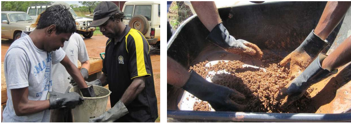
Figure 5. Hand mixing the rock base in a bucket (single rock) or wheelbarrow (batch mix).
