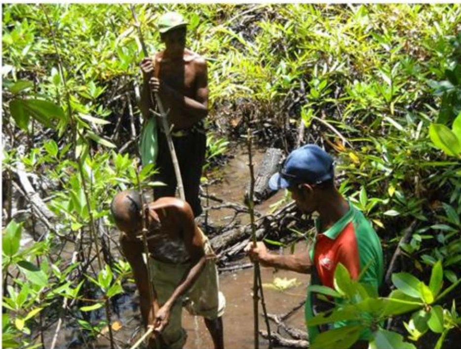
Figure 4. Measuring and marking out of the mud crab mangrove pen at Labubutu.
