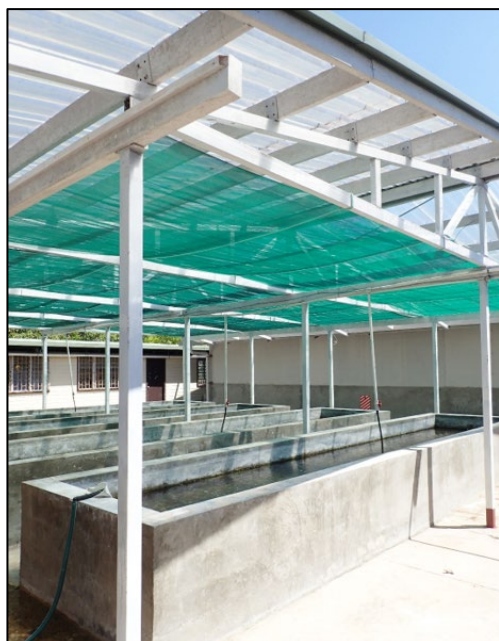
New NIMRF infrastructure supported by the Project – 6,000 L cement raceways and light attenuating shelter
