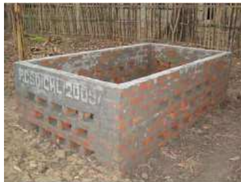
Pic. 10. NADEP composting pit with holes for natural aeration
