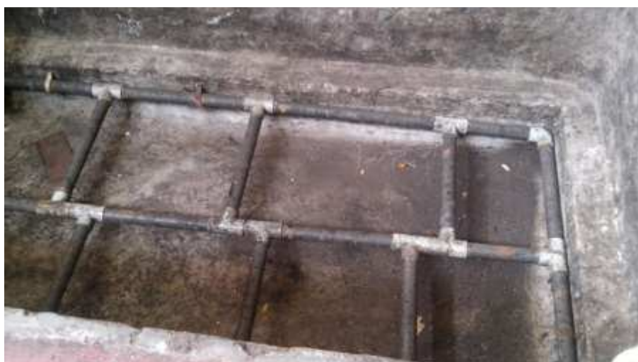
Pic. 3: Bin composting with aeration pipes on the floor of the bin observed in "Kasa to Rasa" Unit- an initiative of the NGO Saahas, Koramangala, Urban Bangalore
