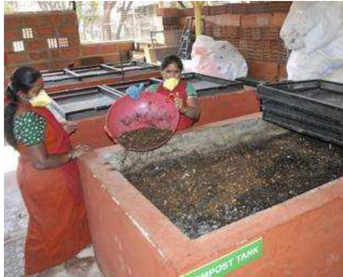
Pic. 13. Staff of Kasa Rasa filling the compost tank for aerobic decomposition of waste
