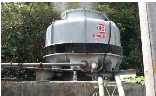
IMAGE 41 A blower reduces the temperature of water flowing into the condensers at Sendangmole cajuput oil distillery, Gunungkidul. Credit: Prastyono
