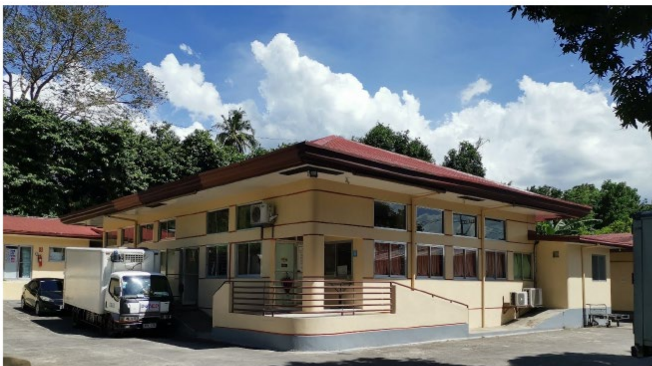
The Kalipunan ng mga Kooperatibang Maggagatas, Inc. (KMMI) Milk Processing Facility and Main Office in Brgy. Lamut 2, Calauan, Laguna visited on May 10, 2022
