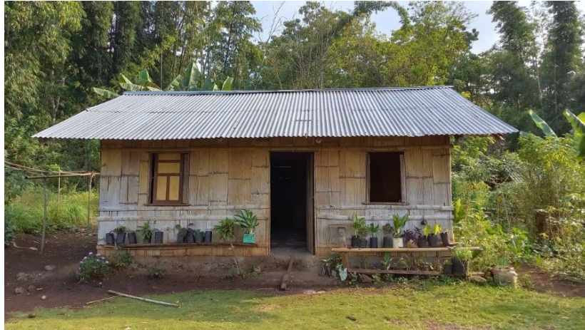
Figure 14 Bamboo-based housing construction made by the communities
