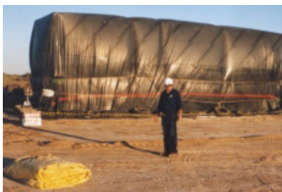
Sheeted fumigation of portable buildings.
