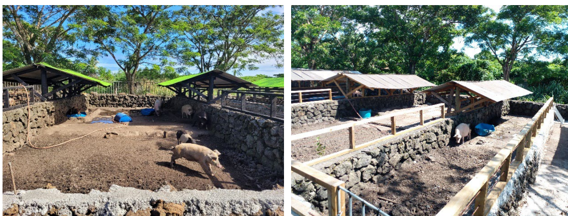
Paradise Taveuni renovated piggery pens.
