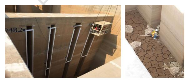
Figure 1. Installation of the PIT antennas to the vertical slots (source: XPCL).
