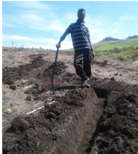
Digging a main drain in a low-clay soil (Source: Rauke Buimeng)
