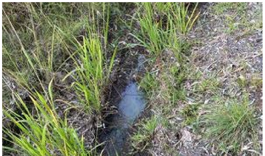
Vegetation blocking drain flow
