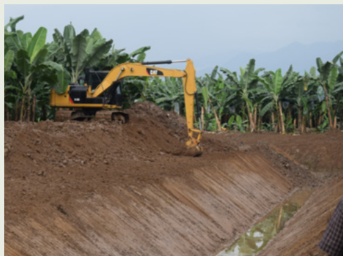
Preventing water from entering the farm via neighbouring farms can reduce the risk of a Fusarium wilt incursion.
