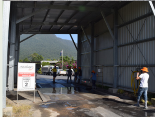
Vehicle washdown facility in the Philippines (above) and a vehicle bath in north Queensland, Australia (below)
