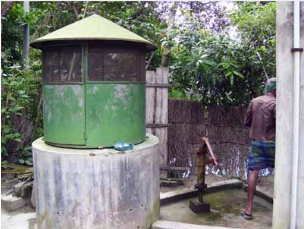
A dug well that provides arsenic-safe water to 200 families
