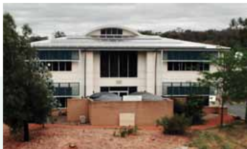
A bank of 48 solar panels was installed on the roof of ACIAR House in Canberra as part of ACIAR's Climate Change Initiative.
