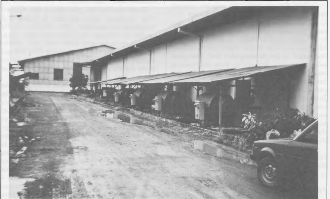
These deep bed drying bins in Malaysia are to have computer controllers fitted to their fans and burners for studies forming part of Project 8308.
