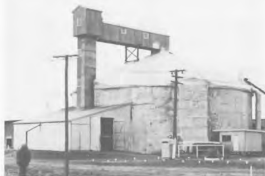
Fig. 8. Grain refrigerated aeration system on an insulated 5400 t squat silo at Brookstead, Queensland.
