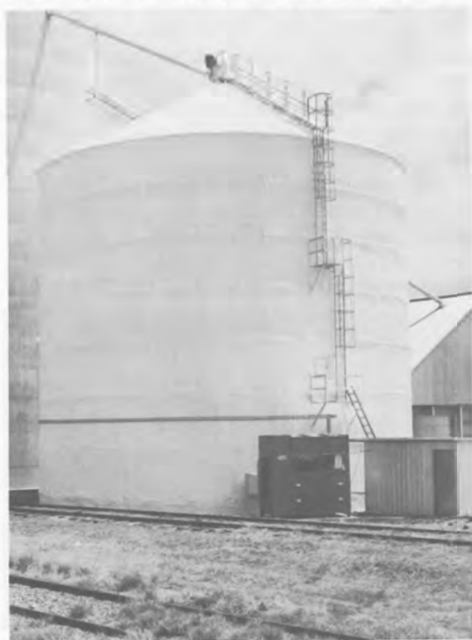
Fig. 10. Refrigerated aeration system on a 1700 t silo at Lah, Victoria.
