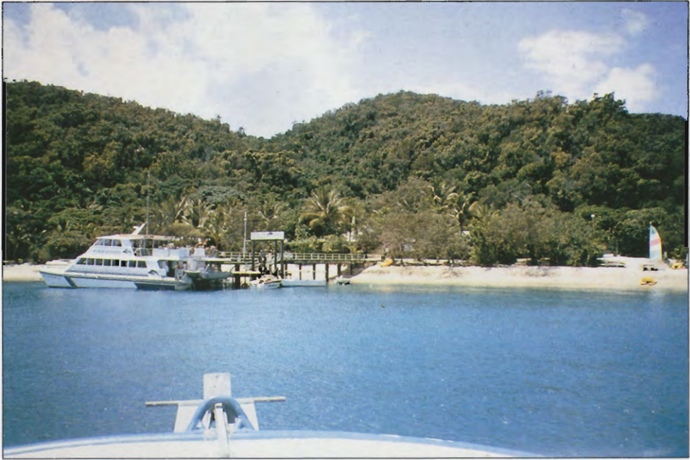
Figure 17.1 Jetty at Fitzroy Island
