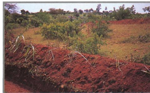
**Newly constructed *fanya juu* terracing: more than 80% of farmers in semi-arid Ukambani protect their land with these contour banks. However, while these banks prevent erosion by controlling rain-water runoff, they do little to help maintain the soil's fertility.**
