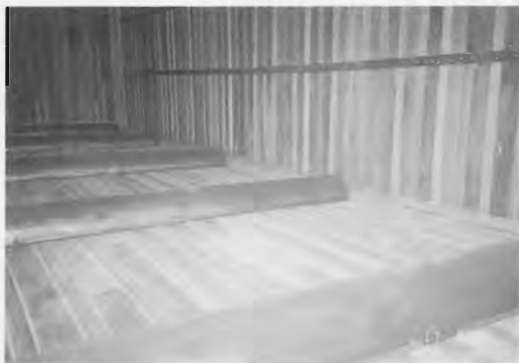
Figure 1. Air ducts in elevated wooden shed.
