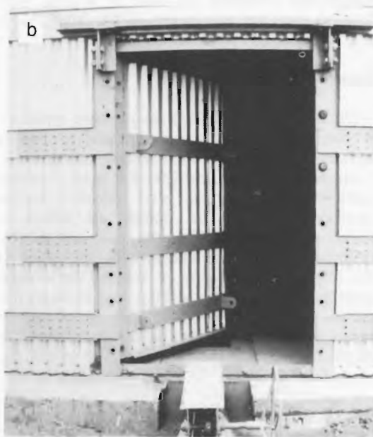
Fig. 13. Machinery access doors: (a) light door with internal louvres; (b) heavy door able to cope with grain pressures and wall stresses.
