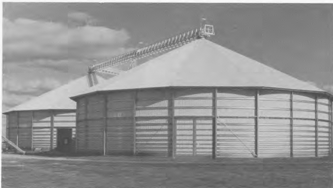
Fig. 9. Gastight bolted light gauge steel silo.
