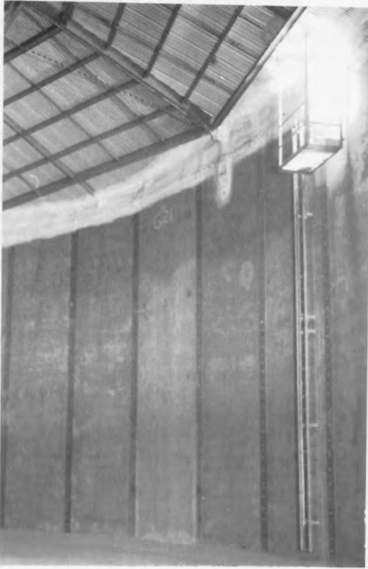
Fig. 10. This figure illustrates the application of polyurethane foam for sealing the joint between the concrete wall and corrugated steel roof of a squat silo.
