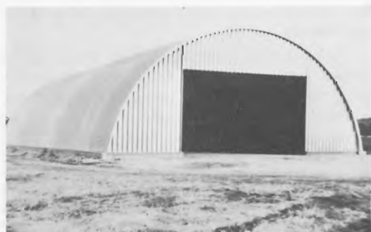
Fig. 7. An arch shed for grain storage, made from deeply corrugated, light-gauge, galvanised steel sheeting.
