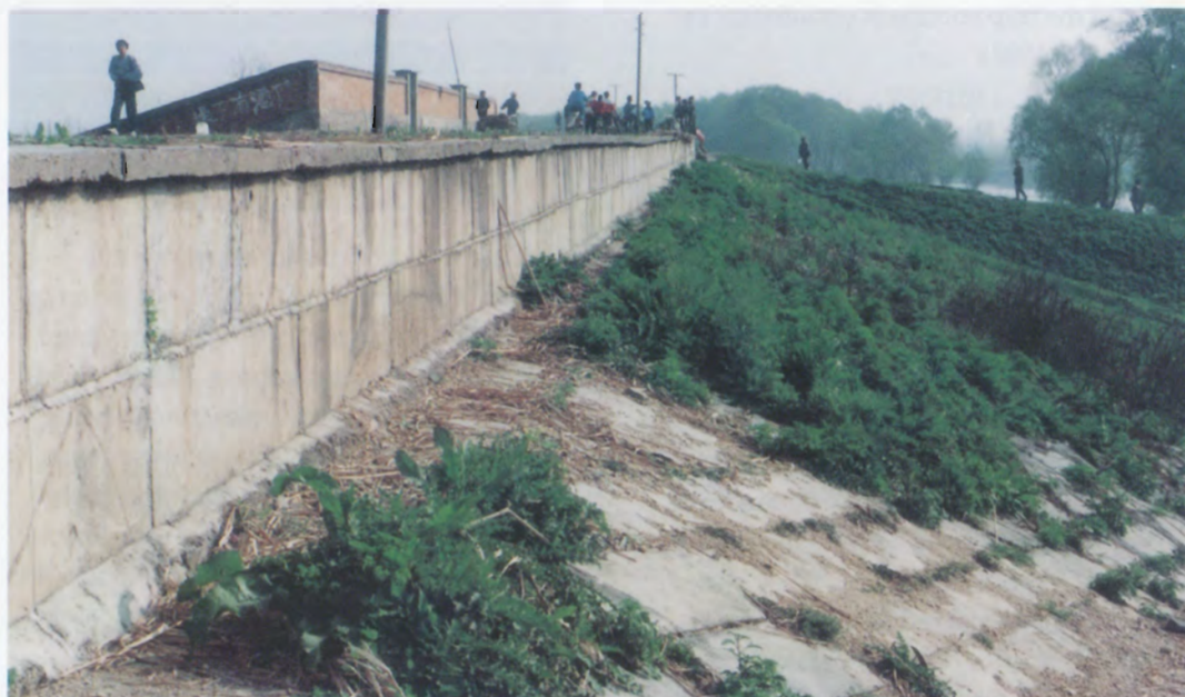
Figure 7. The modified dyke-barrier system for controlling oriental voles.
